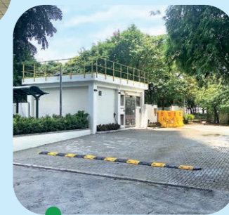
開放毗鄰鴨脷洲大街污水泵房的圍封地方 Opening up an enclosed area adjoining ALC Main Street Sewage Pumping Station
