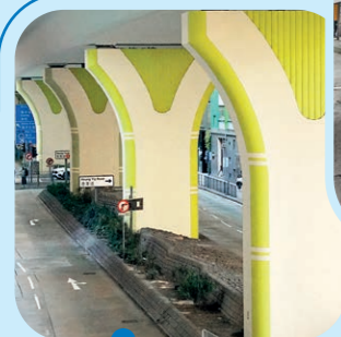
黃竹坑道行車天橋重新掃漆 Repainting of WCH Road flyover
