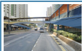
美化香港仔海傍道行人天橋 Facelifting of footbridge at Aberdeen Praya Road
